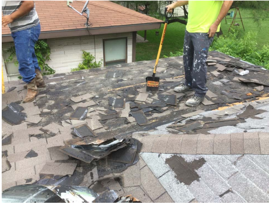
Fig. 2: Installation of new high-solar reflectance, cool, roofs
